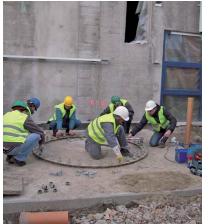
Disassembly of the centering ring for the foundation basket
