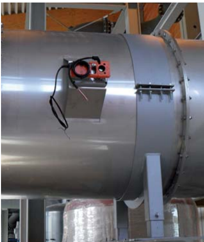
Fixed-point in the interior area in S235, ground and coated
