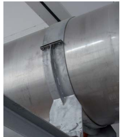
Fixed-point in the exterior area in S235, hot-dip galvanized
