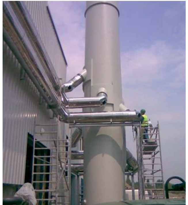
Finished chimney incl. connecting line Jeremias DW-KL
