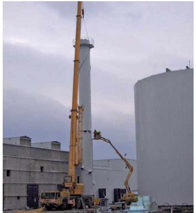
The 6 internal pipes are connected / flanged
