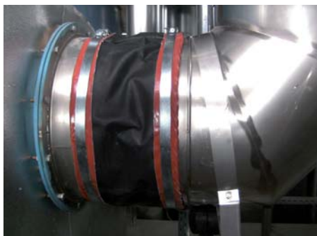
Mesh compensator with clamp
