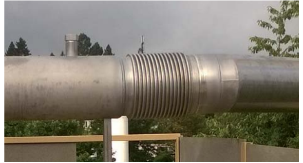
Stainless steel compensators for welding
