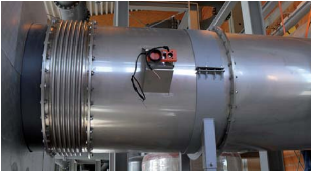
Stainless steel compensators for flanging
