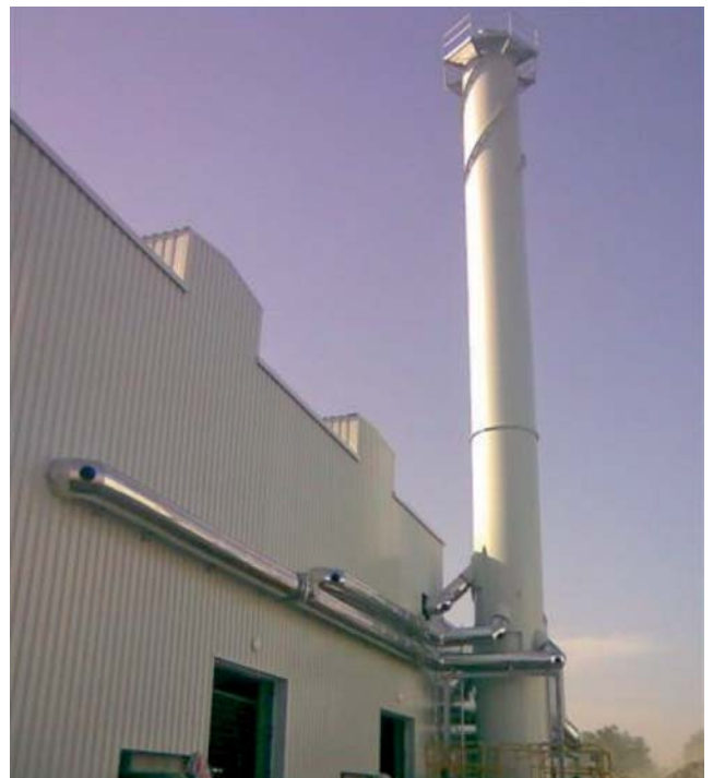
Finished chimney incl. connecting line Jeremias DW-KL
