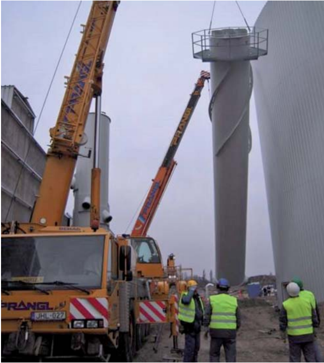
Lifting the upper section with main and revision crane
