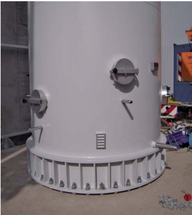
Affix the lower chimney section
