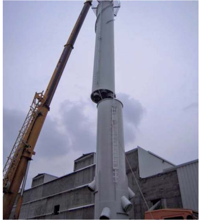
Placing the second section
