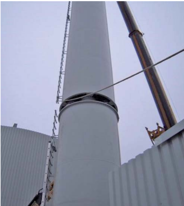
The 6 internal pipes are connected / flanged
