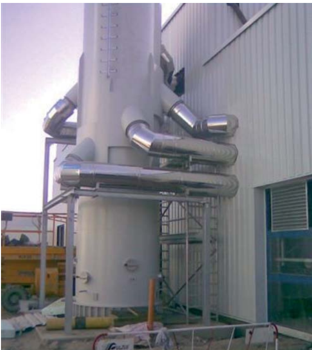
Finished chimney incl. connecting line Jeremias DW-KL
