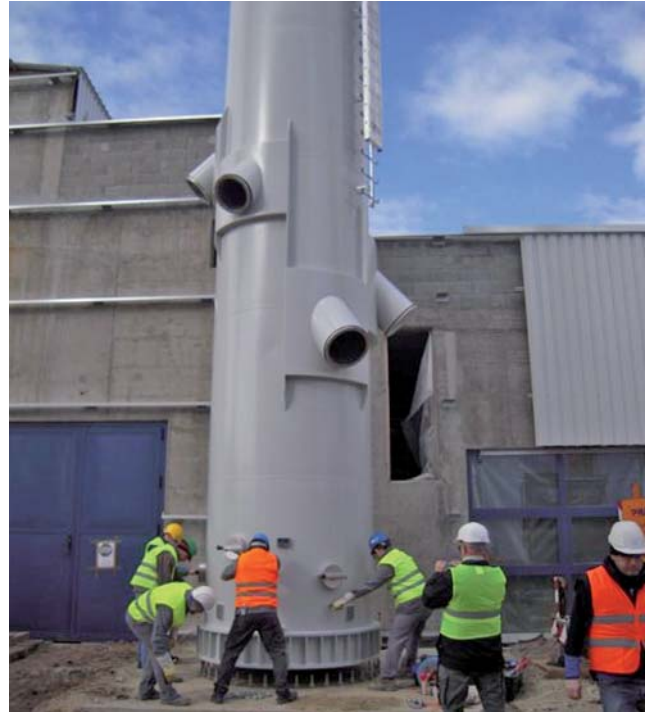
Position the lower chimney section on the foundation basket
