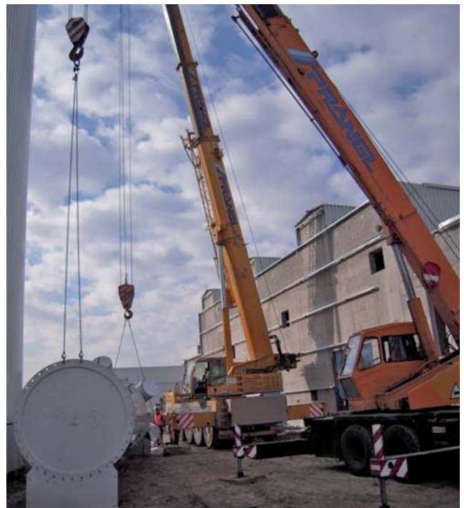
Auto-crane ready for transport
