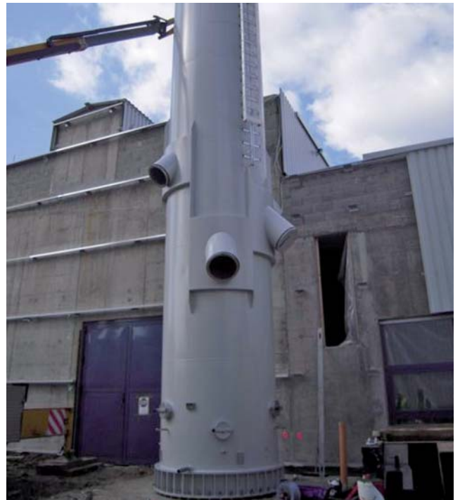
Position the work platform for installing the upper section
