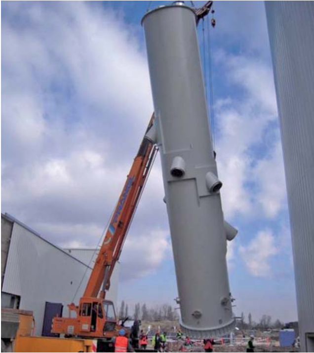
Lifting the lower chimney section
