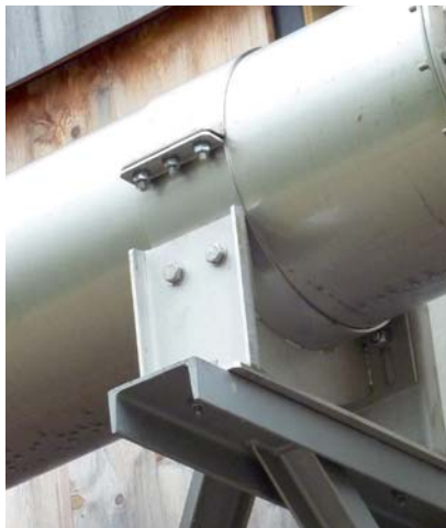
Fixed-point in the exterior area in stainless steel 1.4301
