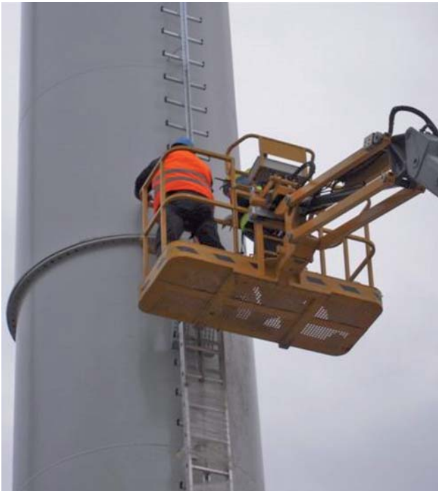
Supporting pipe is screwed on
