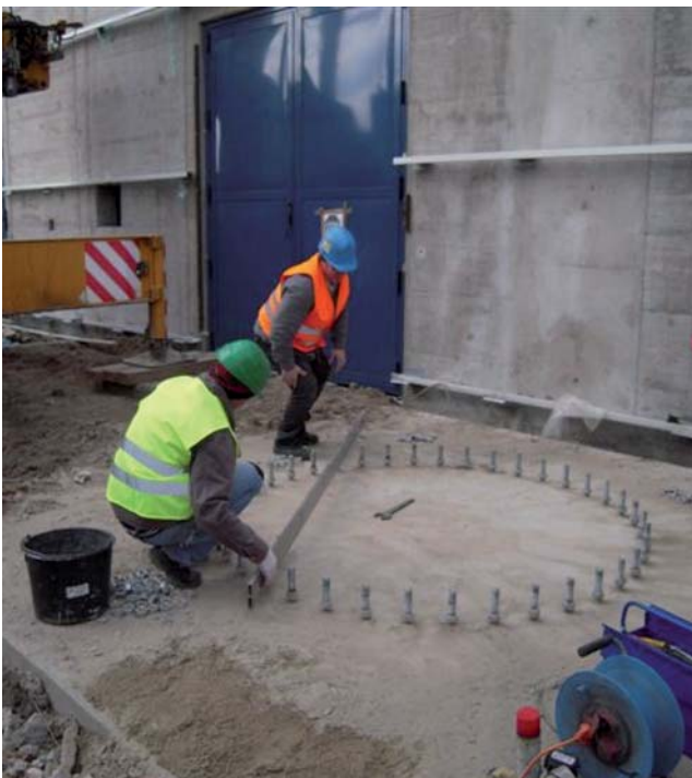
Setting up the anchor nuts 1
